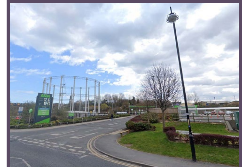
View looking towards gas storage chamber adjacent to Oyster Street car park
