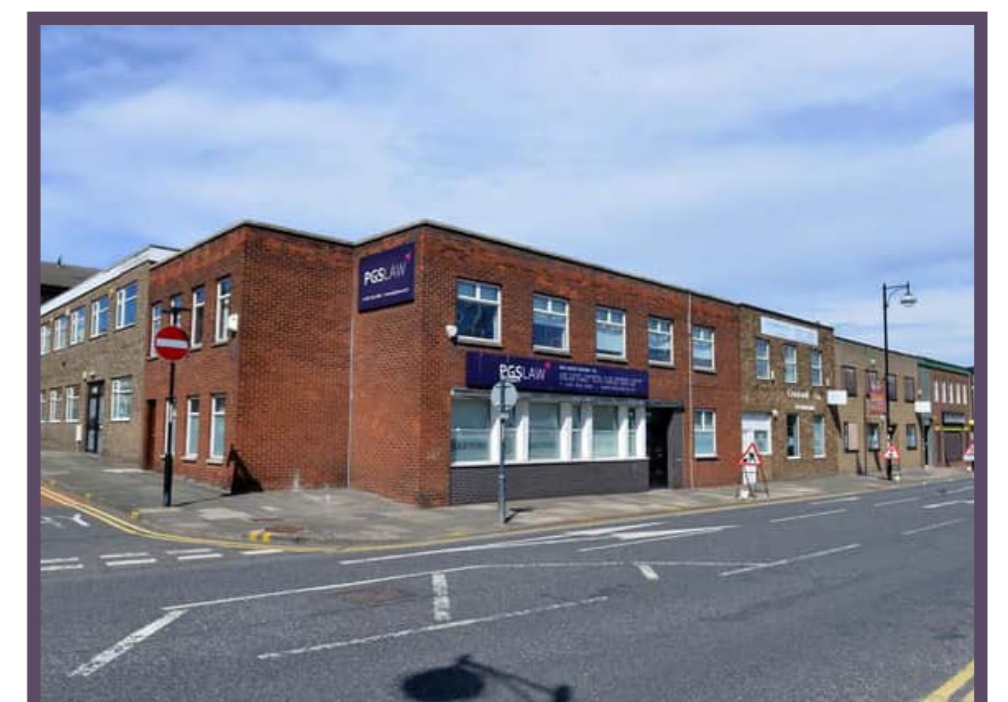
Office buildings on northern side of Coronation Street to be demolished as part of Tyne Coast College Campus
